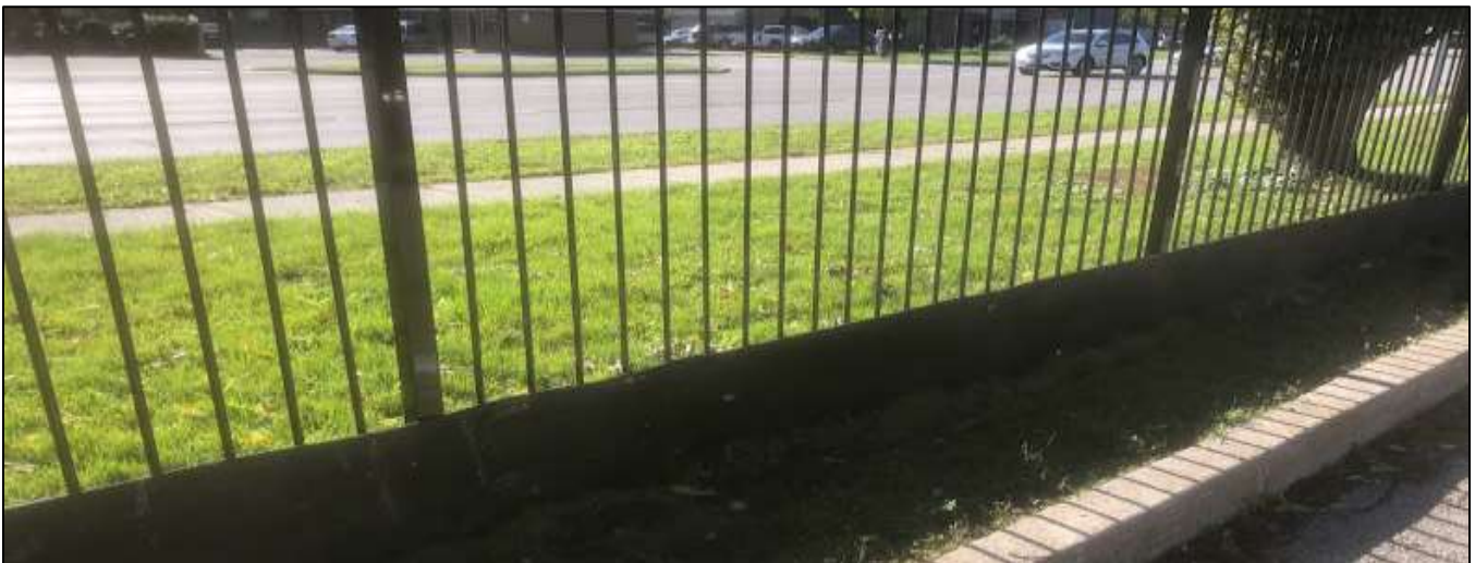
Figure 37 Roadkill mitigation small animal fence, ongoing installation at Cootes Paradise and Grindstone Marsh.
